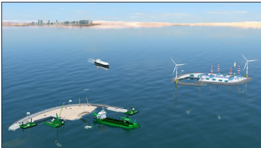
Artists impression of the artificial islands being constructed for the Satah al-Razboot (SARB) offshore oil field
