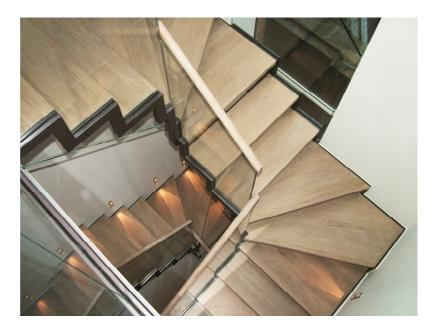
A pre-manufacture sample showing the connection between glass, timber and steel without any visible fixings was able to satisfy everyone and secure the deal.
