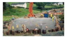
The County Engineers departed from this guidance in determining to use stainless reinforcement throughout the structure.
