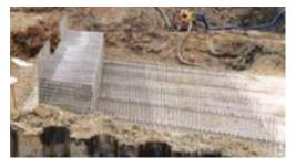
The Engineers also took into consideration the forgiving qualities of stainless steel. The concern about accurate translation of what is designed and specified in an office to actual practice on site can lead, for example, to lower than expected cover. A non-corroding form of reinforcement absorbs such variations thus avoiding future maintenance concerns.
